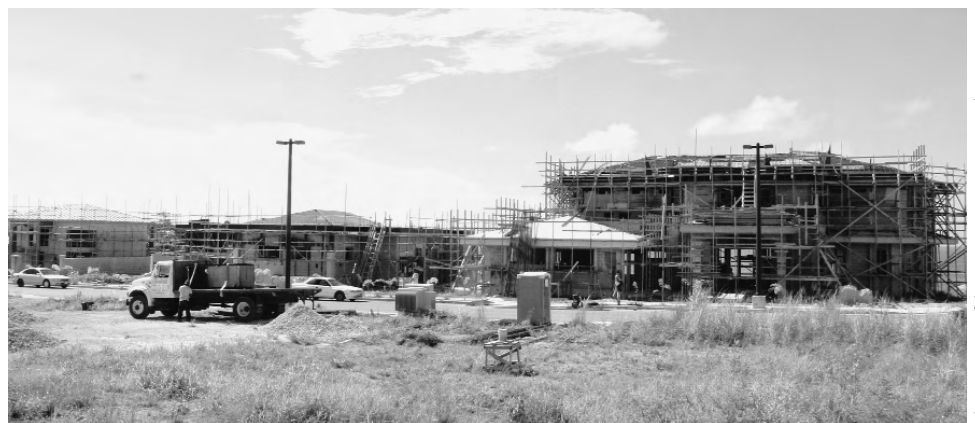
Stella Vista Estates construction in Maite, Guam.
